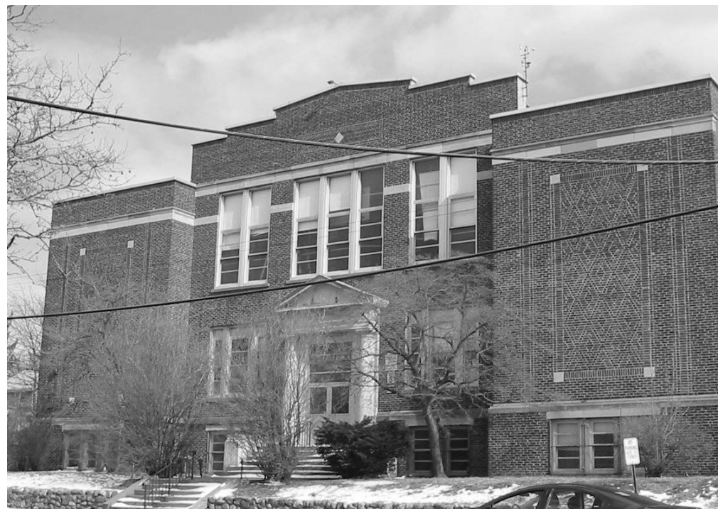
The Dewey school will be soon be replaced with senior housing. It is fitting that a school which once educated our senior citizens will now house them, affording them an opportunity to remain in the the community in which they have spent their lives.
