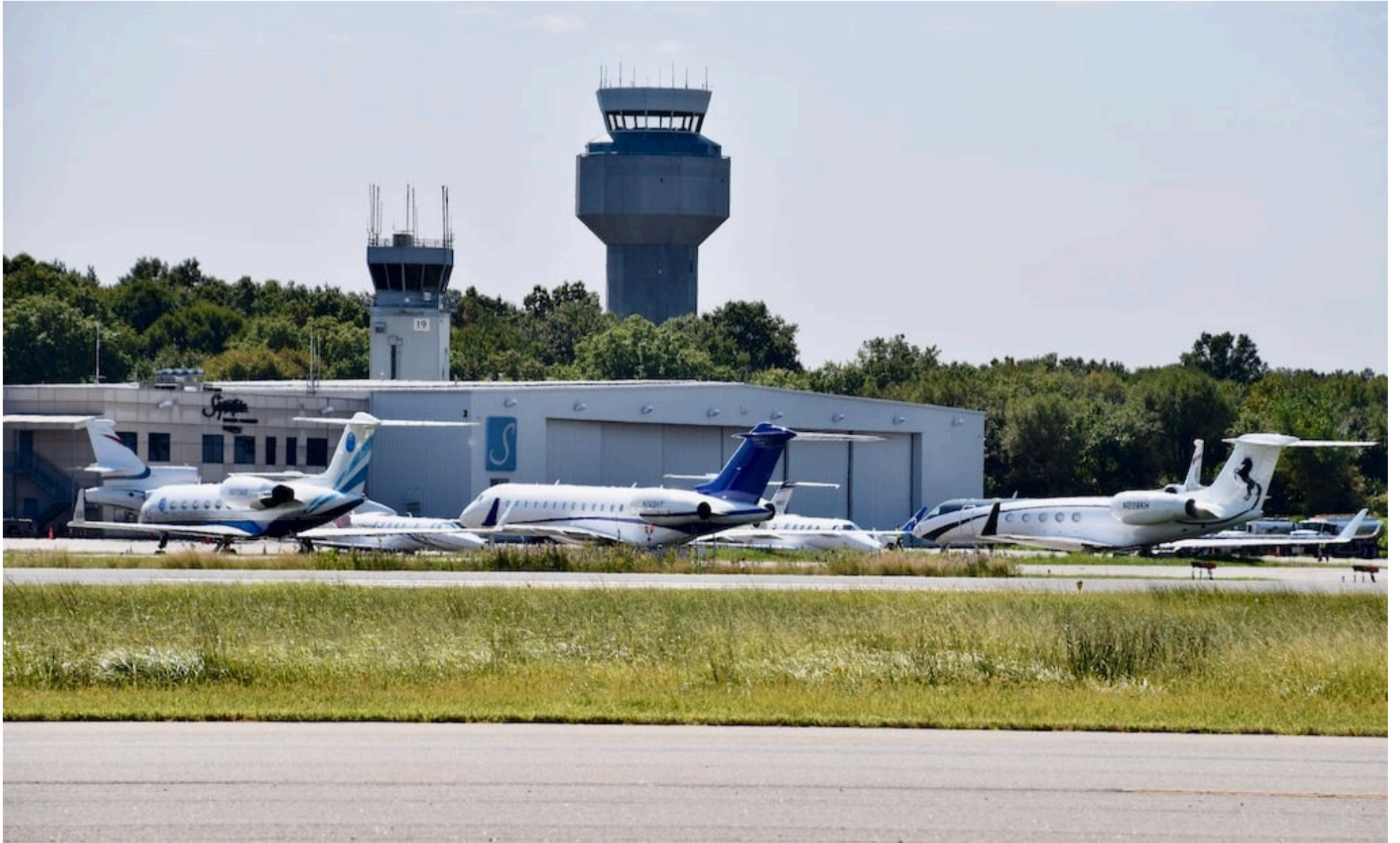
The FAA's new ATC tower overlooks the existing tower at Teterboro Airport. Credit: Bill Carey
